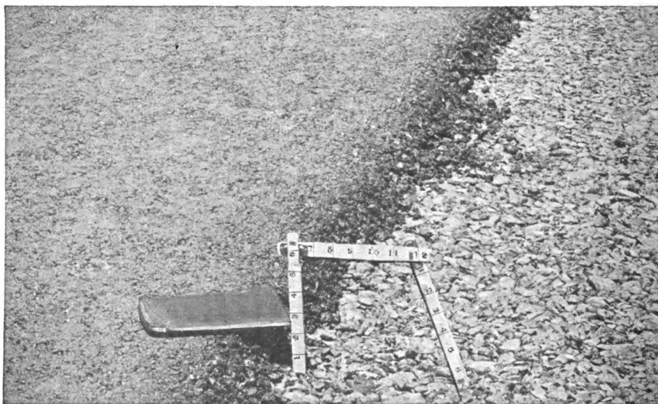
Figure 115. A 2-inch compacted hot-mix pavement on crushed rock base.
